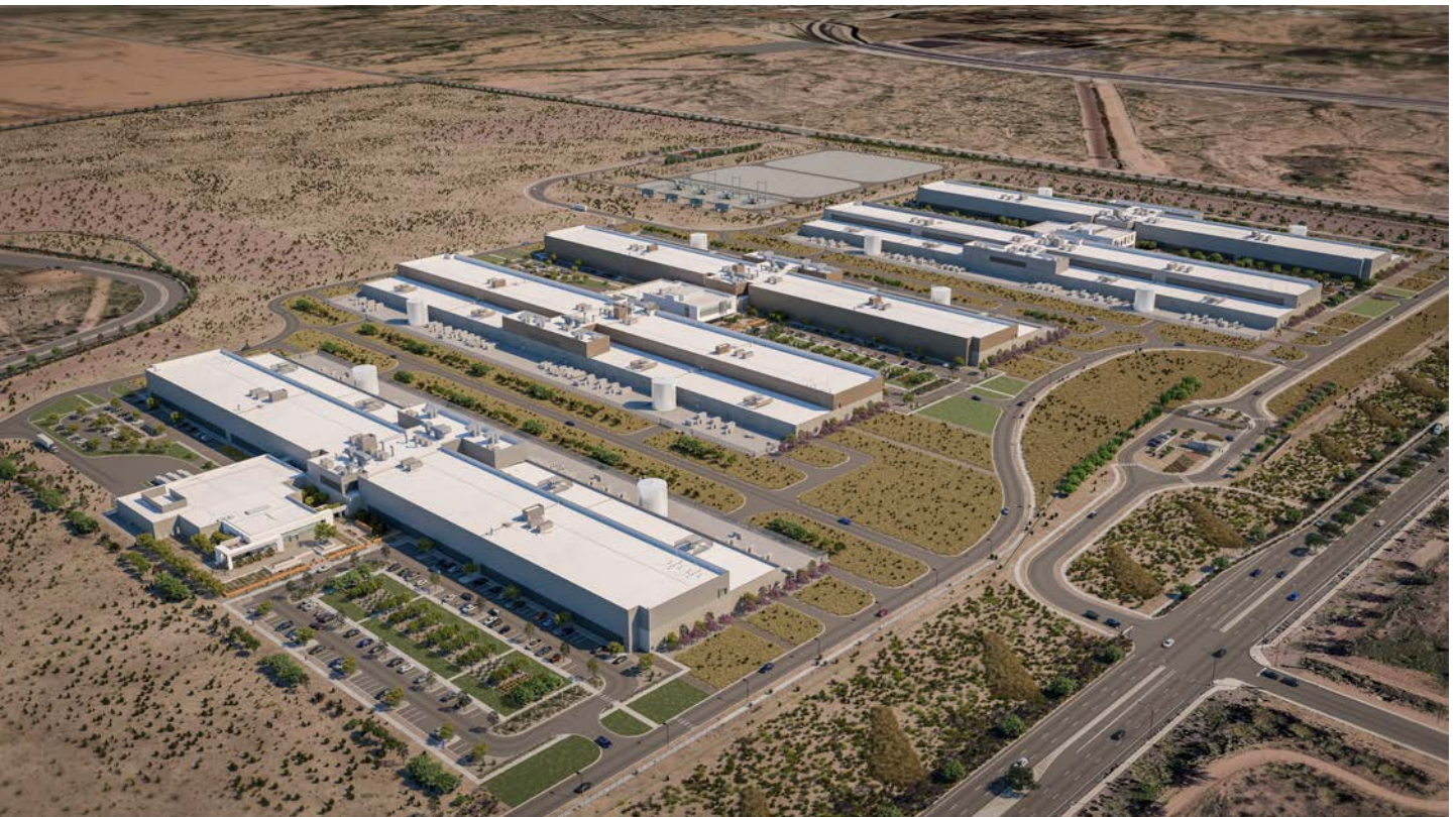
Above: Meta announced it is expanding the Meta Mesa Data Center with three new buildings. The campus, which was first announced in August 2021, will now include five buildings totaling more than 2.5 million square feet.
